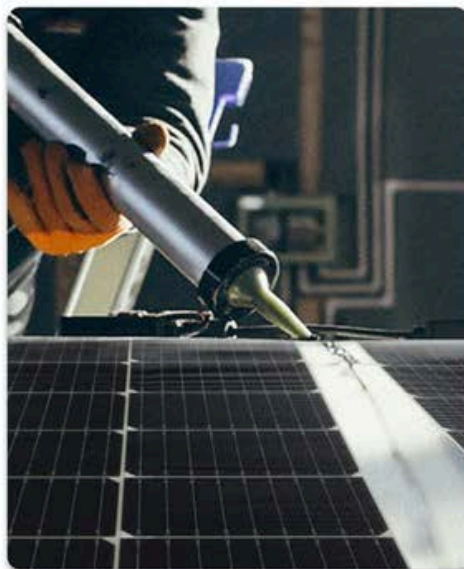
Drill-Free Installation Using Silicone Adhesive
